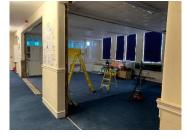
The work started on the first day of the school holiday where the internal classroom partitions glazing and doors were replaced. At one point in the holiday, school was looking rather 'open plan' with the walls and partition walls all taken down. In addition new fire detection and emergency lighting has been installed along with a brand new fire alarm system.
